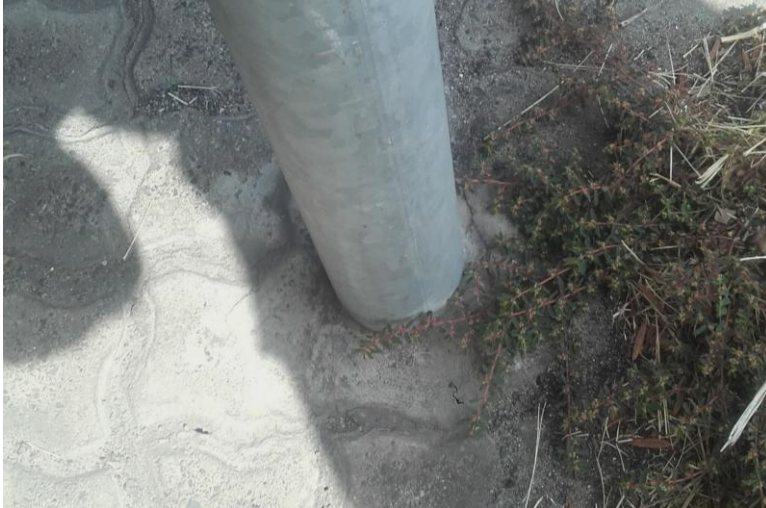
Fig 3.3 Post base to be cast flush with existing surface level
