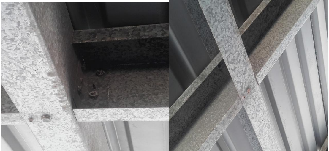
Fig 3.5 Typical bearer and purlin connection
