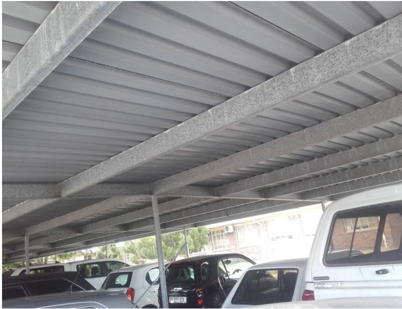
Fig 3.7 Typical posts, bearers and purlins configuration
