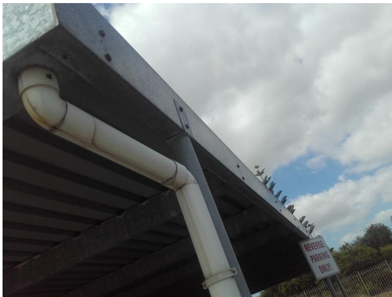
Fig 3.6 Typical down pipe and gutter connection
